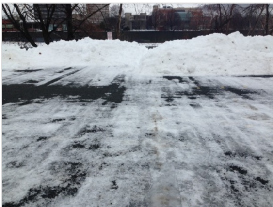
Figure 2: A TRUEGRID Surface immediately after plowing.
